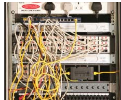
A Furse ESP Cat-5e/Gigabit (left and detail below) protecting a hub from transient overvoltages on a network connection with another building
