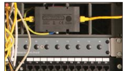
A Furse ESP Cat-5e/Gigabit (left and detail below) protecting a hub from transient overvoltages on a network connection with another building
